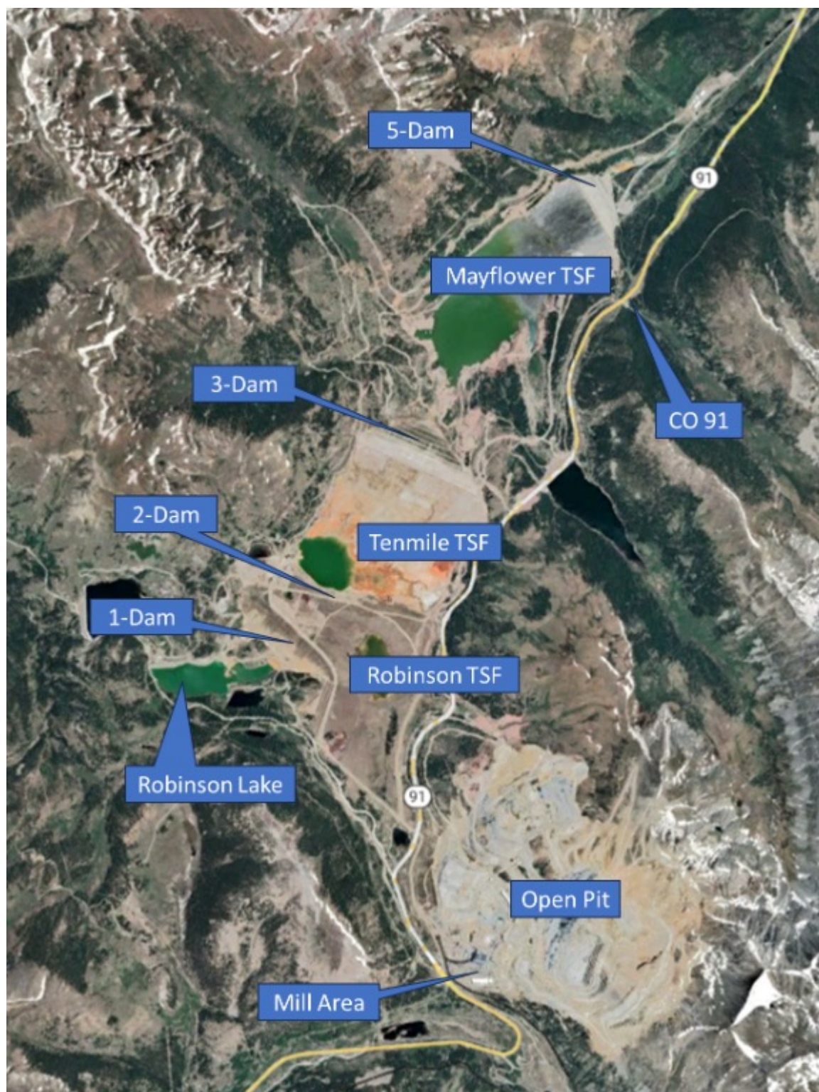
Figure 3. General Climax Mine Layout (Imagery from October 2024).
